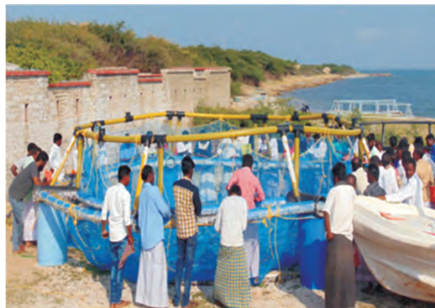
A Cage is getting ready for installation
